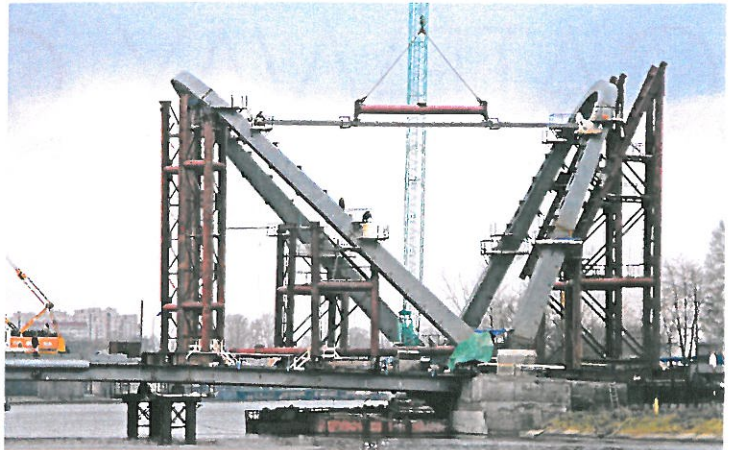
The bridge under construction showing temporary supports
